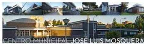
CENTRO MUNICIPAL JOSÉ LUIS MOSQUERA
